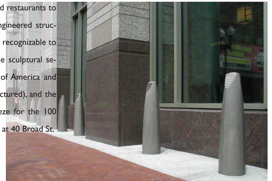
Cast stainless steel security bollards fabricated and installed by Make Metals Ltd. at the State Street Financial Center.
