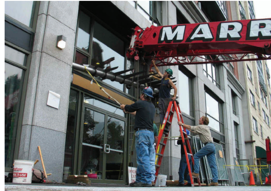
Installation of structural awning component, at the Grandview Residences on Tremont St, to later be covered with laminated glazing for architect and client, Jung Brannen.
